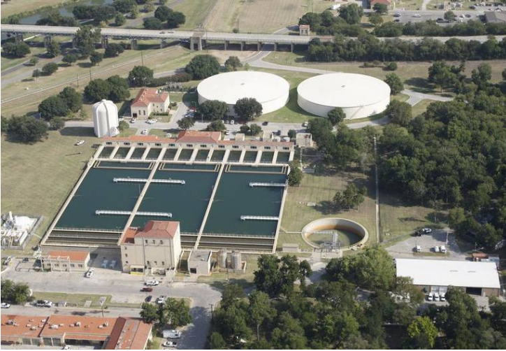
Fort Worth's Holly Water Treatment Plant west of downtown. Ron T. Ennis - Star-Telegram archives
